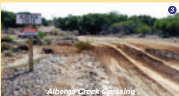
Alberga Creek Crossing
