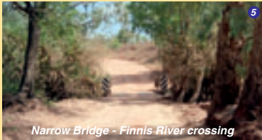
Narrow Bridge - Finnis River crossing
