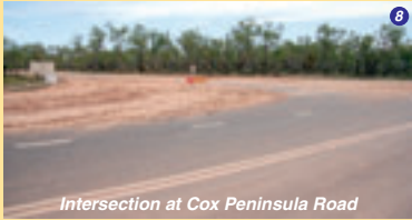
Intersection at Cox Peninsula Road
