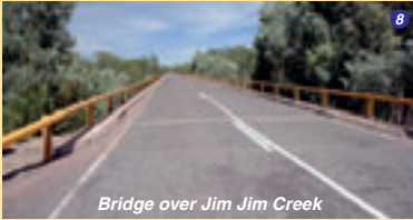
Bridge over Jim Jim Creek
